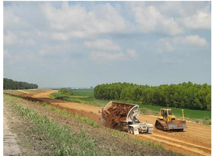
Figure 1: Levee Restoration in progress
